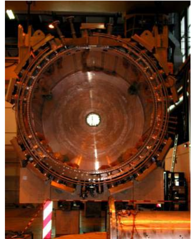
ECC rotated with all feedthroughs installed, Mar 2003
