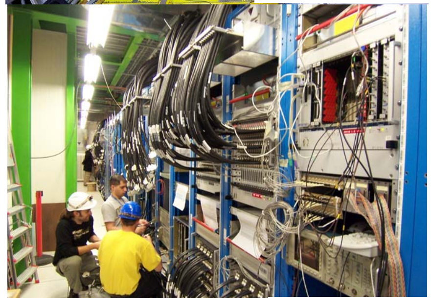
LVL trigger cabling
