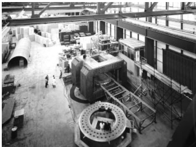
Fig. 1.3: Installing the coils.
