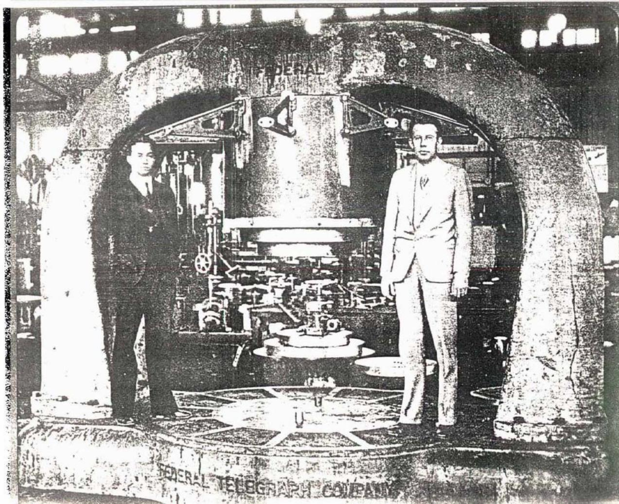
Livingston and Lawrence with the magnet of the “27-inch” (later “37-inch”) cyclotron on which most of Berkeley’s 1930s nuclear physics was performed.
