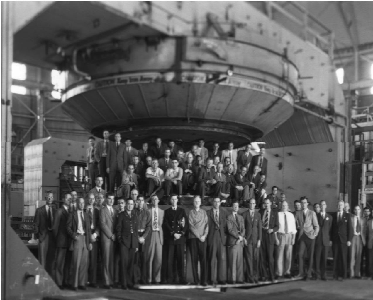
The Berkeley 184" was begun in 1939 as a classical cyclotron, to be operated with  $V_{rf} = 1$  MV, but WWII interrupted rf installation and it was used to test mass spectrographic separation of uranium isotopes. **FM rf was installed in 1946**, yielding **190 MeV d+** (700 MeV p in 1959).
