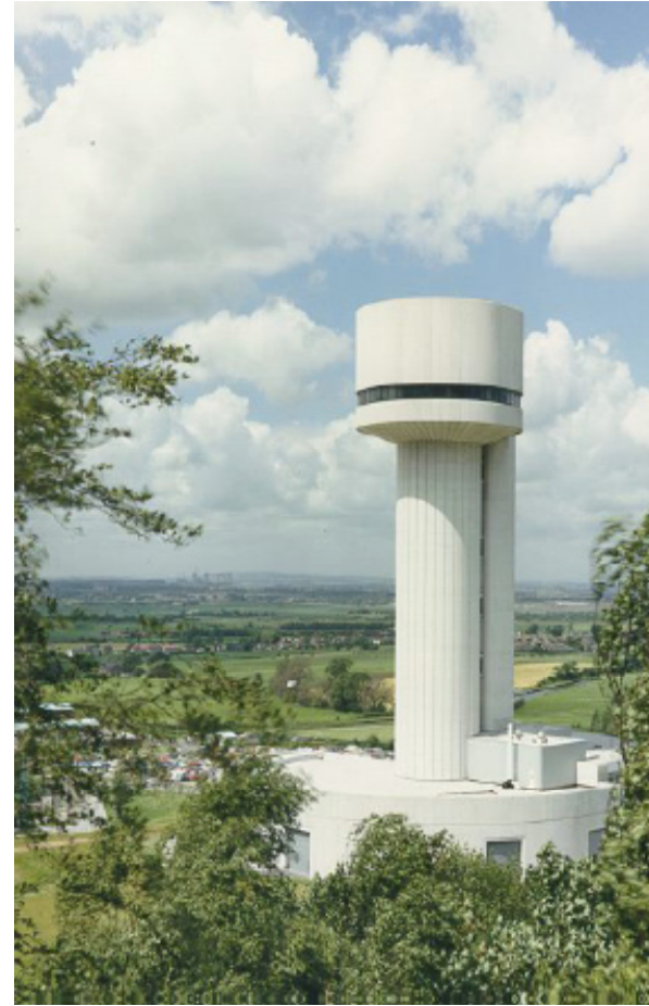
Daresbury folded tandem (20 MV in a 230-ft tower).
